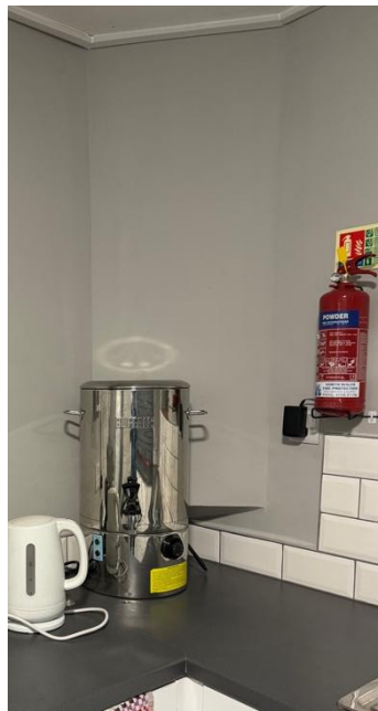
Fire extinguisher in kitchen
