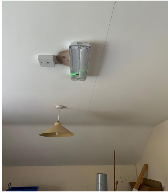
Emergency lighting and fire alarm bell situated in upstairs store room
